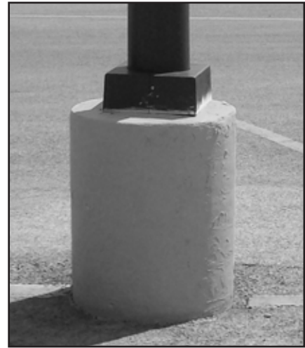
Level the ground around the base
