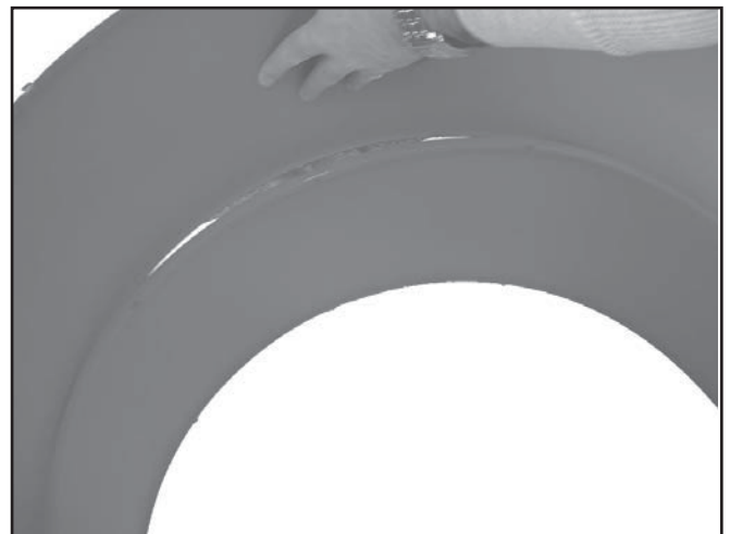
Work the horizontal seams together
